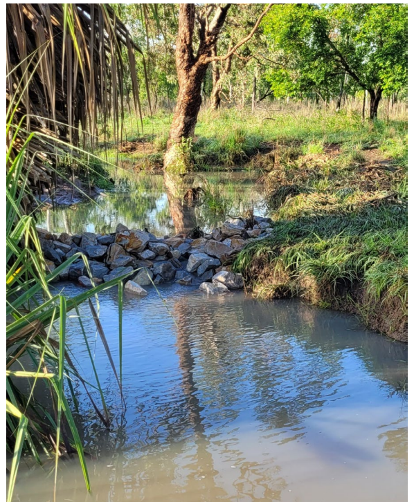
Leaky weirs help rehydrate the landscape on Old Cameron Downs
